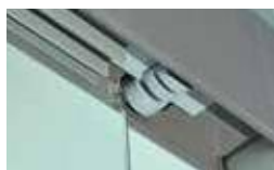
2 Sensors for detector of sash position
